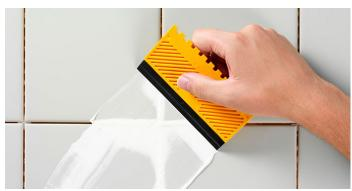
For tiles larger than 250 x 300mm a cement based powder adhesive, such as Bond It CTA FLEXIBLE, should be used. Open time of the exposed adhesive bed is approx 15 minutes, dependant on conditions. Do not apply more than will be used during this period.
